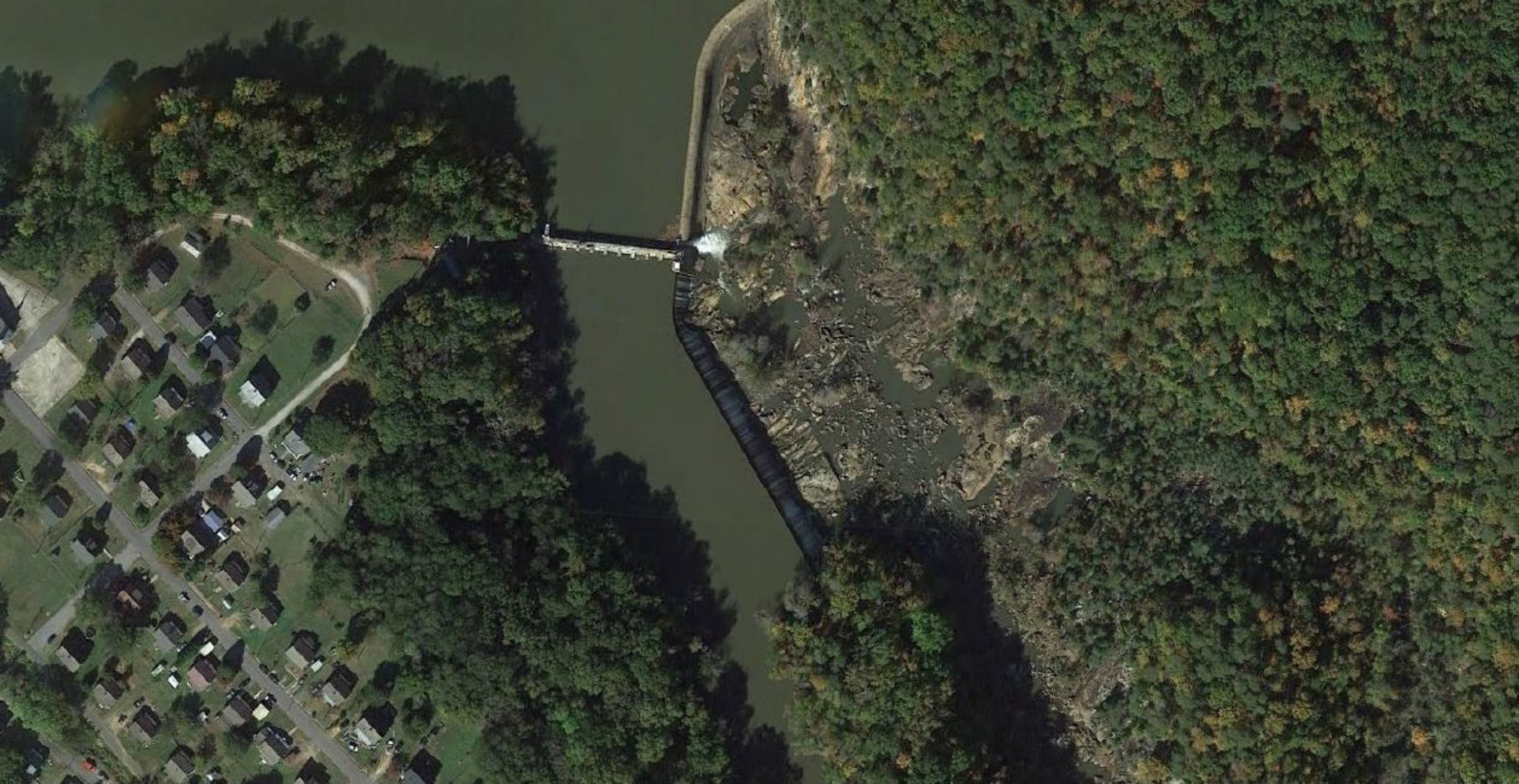
Great Falls-Dearborn Headworks Spillway, Great Falls, SC
