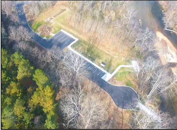
Corpening Bridge Access Area Johns River
