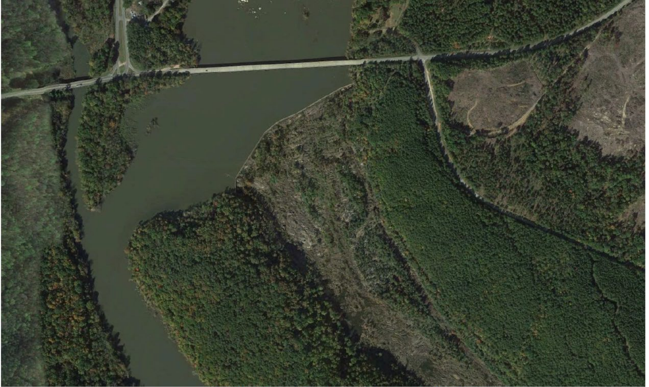
Great Falls Diversion Dam, Great Falls, SC
