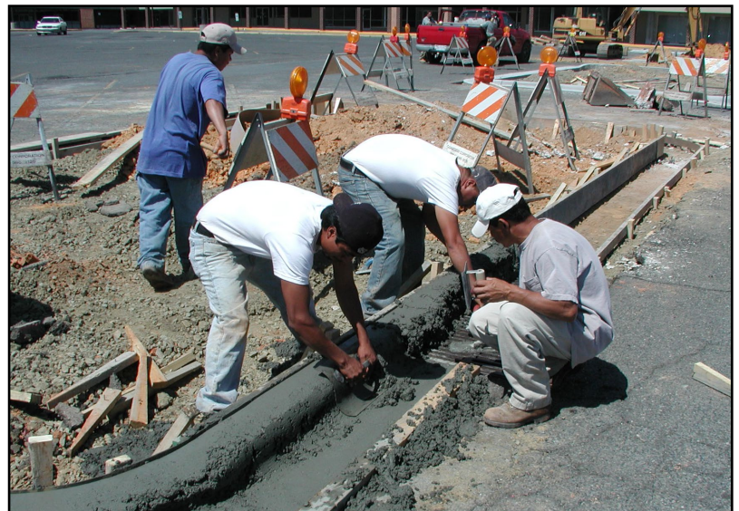
Northcross Retrofit in Huntersville
