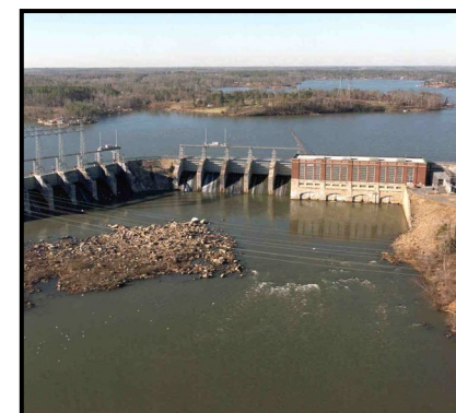
Wylie Hydro Station
