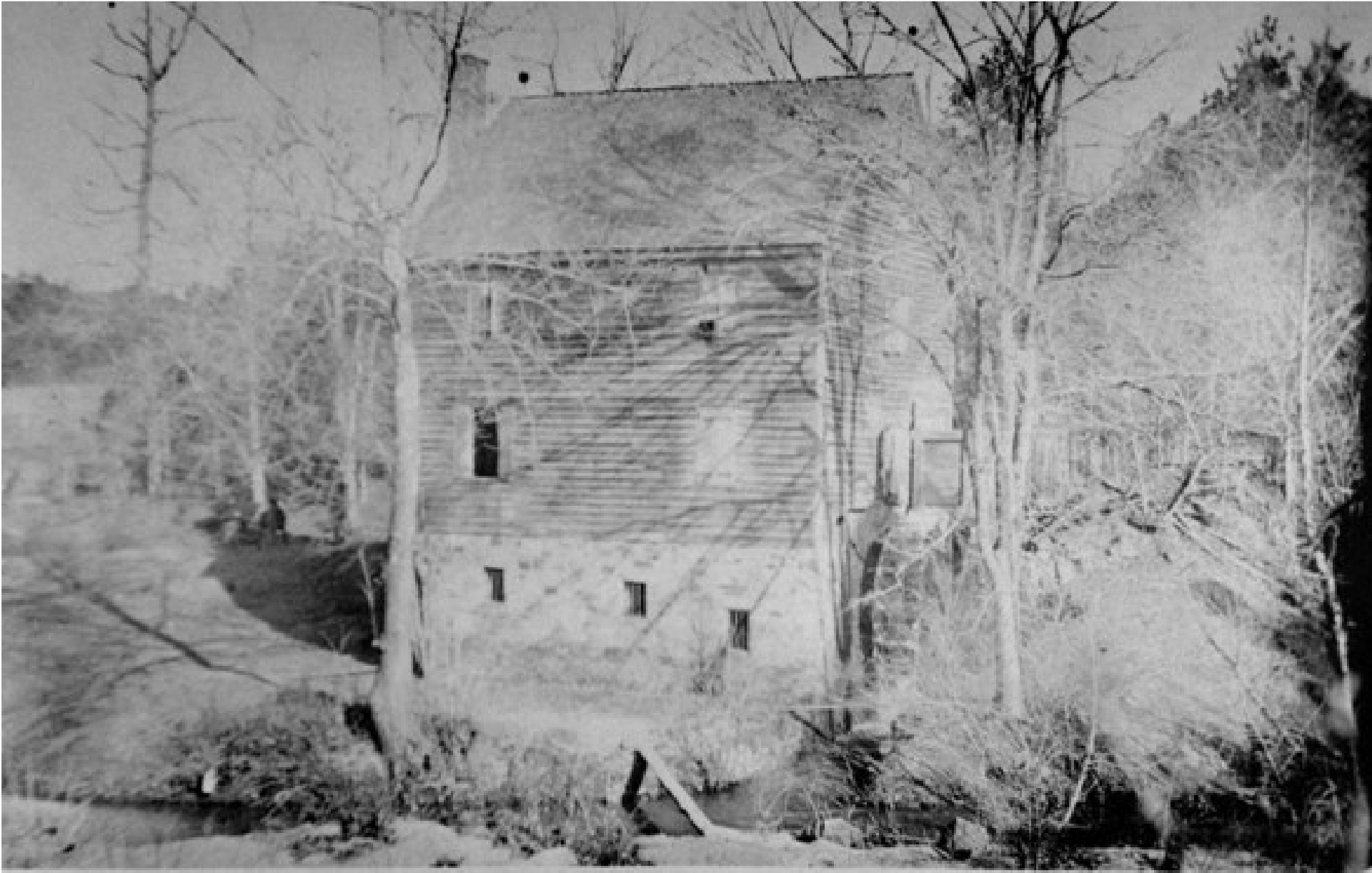
Whitley Mill on Long Creek In Charlotte - 1820 to 1919
