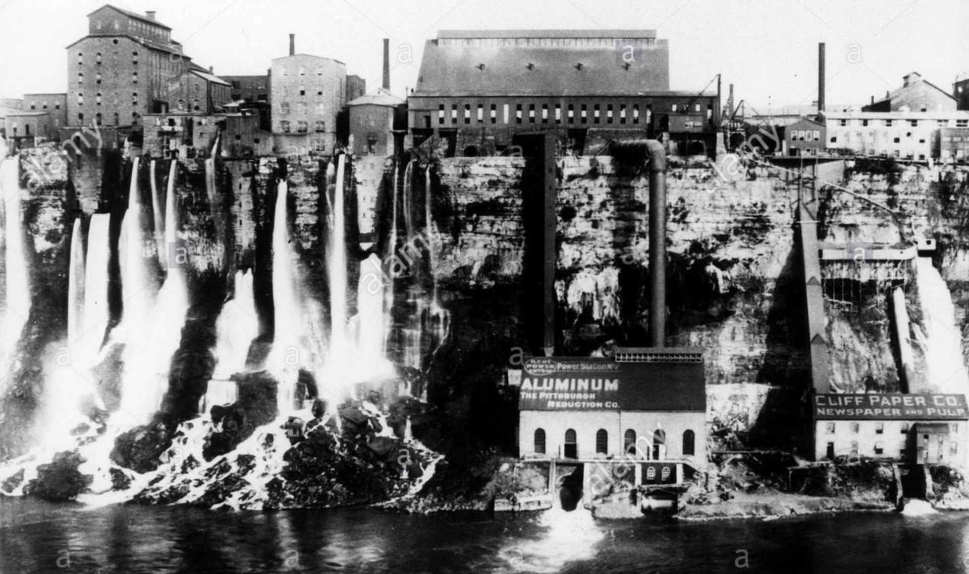
Niagara Falls Hydro Station - 1895
