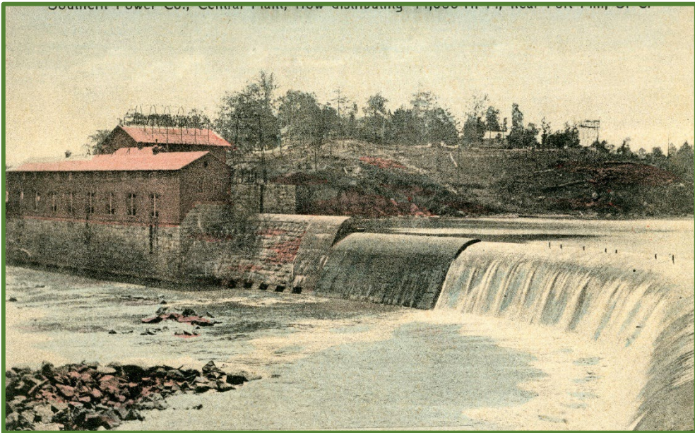
Original Catawba Dam - 1904
